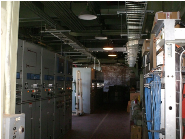
Motor control area before project
