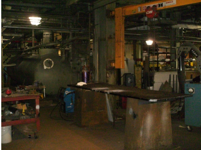
Machine shop before project
