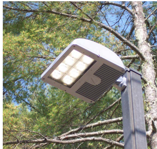
Yard lighting after project
